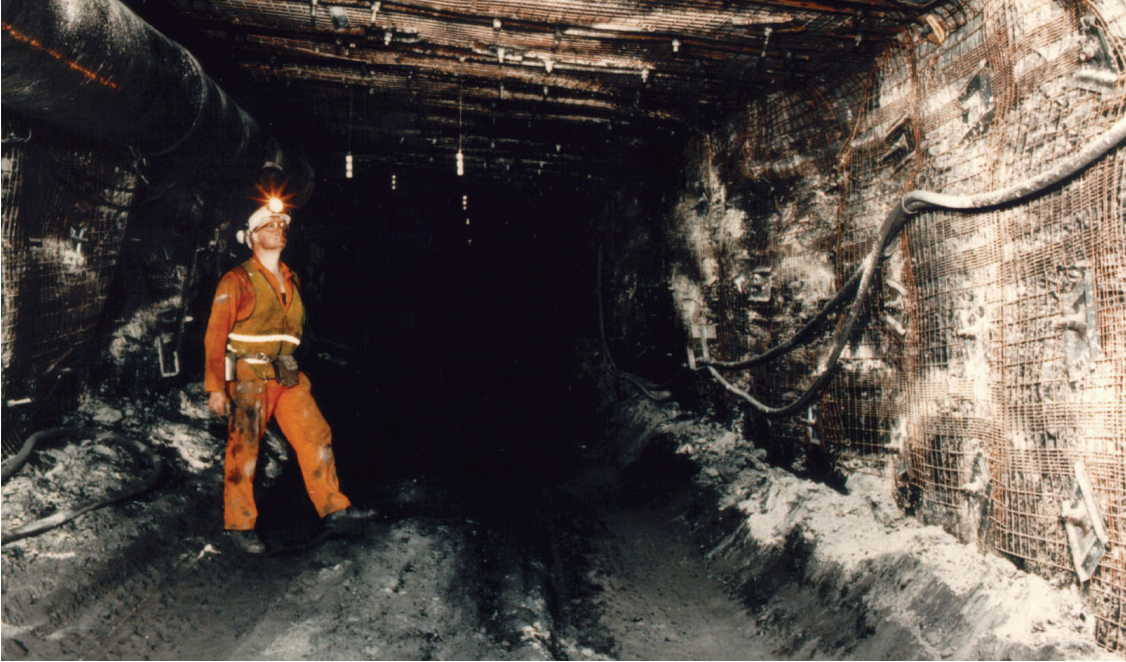
A typical rockbolted roadway.
